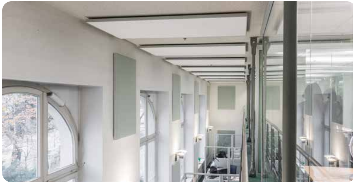
From above: Ceiling absorber with individual connection to the supporting profiles of the industrial ceiling, suspended between lighting levels and system ceiling, in direct mounting with a construction clearance
